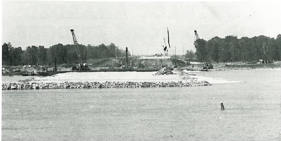
East Belt Freeway – Arkansas River Bridge Approach
